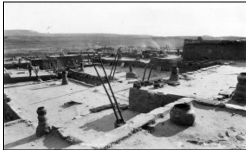
Across the roofs of Zuni
